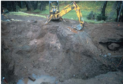
Excavating contaminated soil from Mt. Hood’s Meadows, photo by Kate McCarthy
